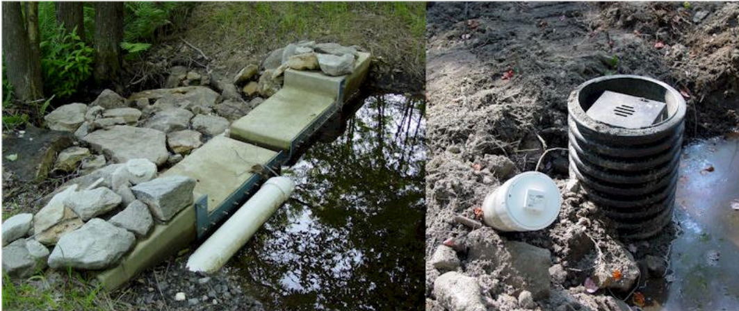
Figure 5 – Typical Check Dam and Agridrain Installations
